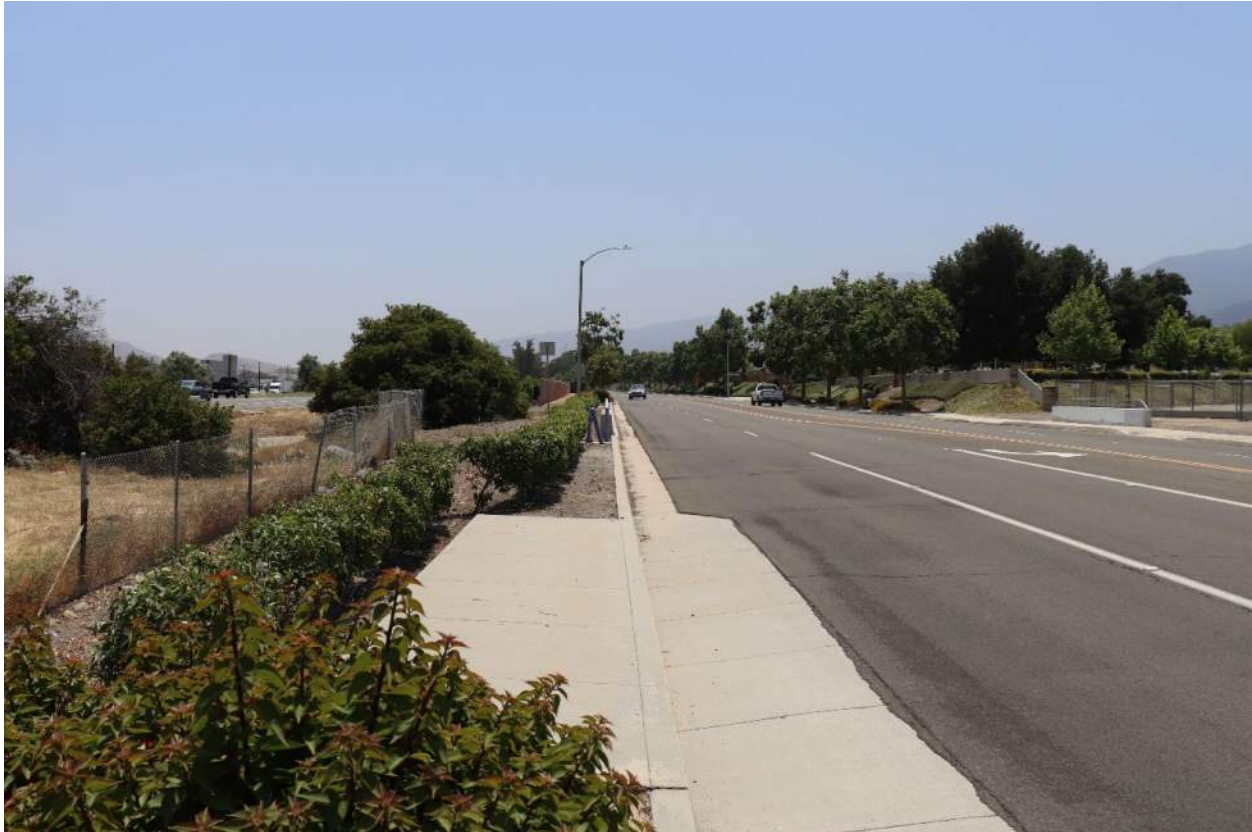
Figure 17. KV-4 Existing Condition
