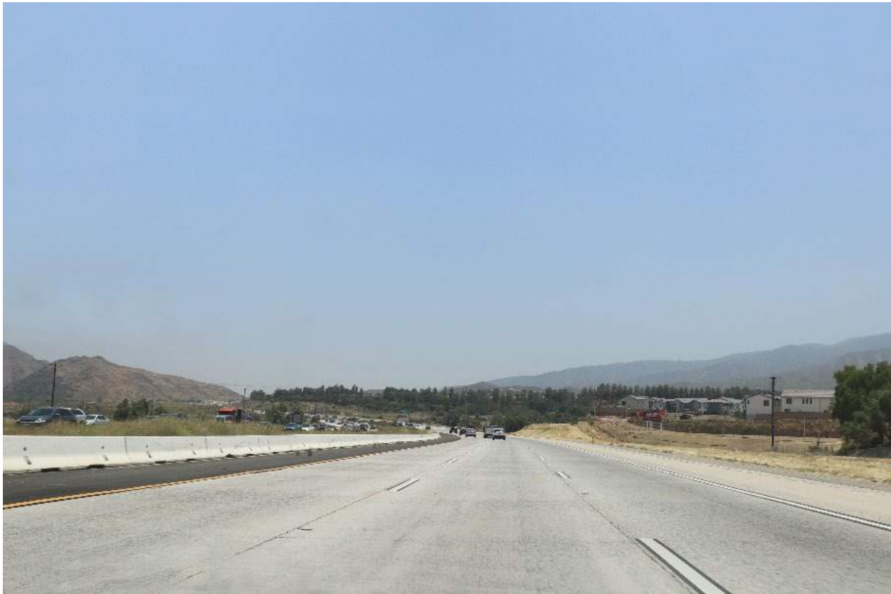
Figure 16a. KV-3b Existing Condition
