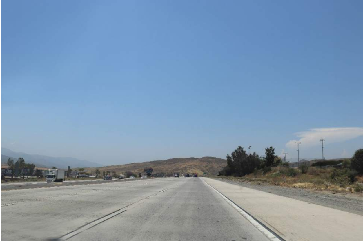
Figure 11. KV-1 Existing Condition
