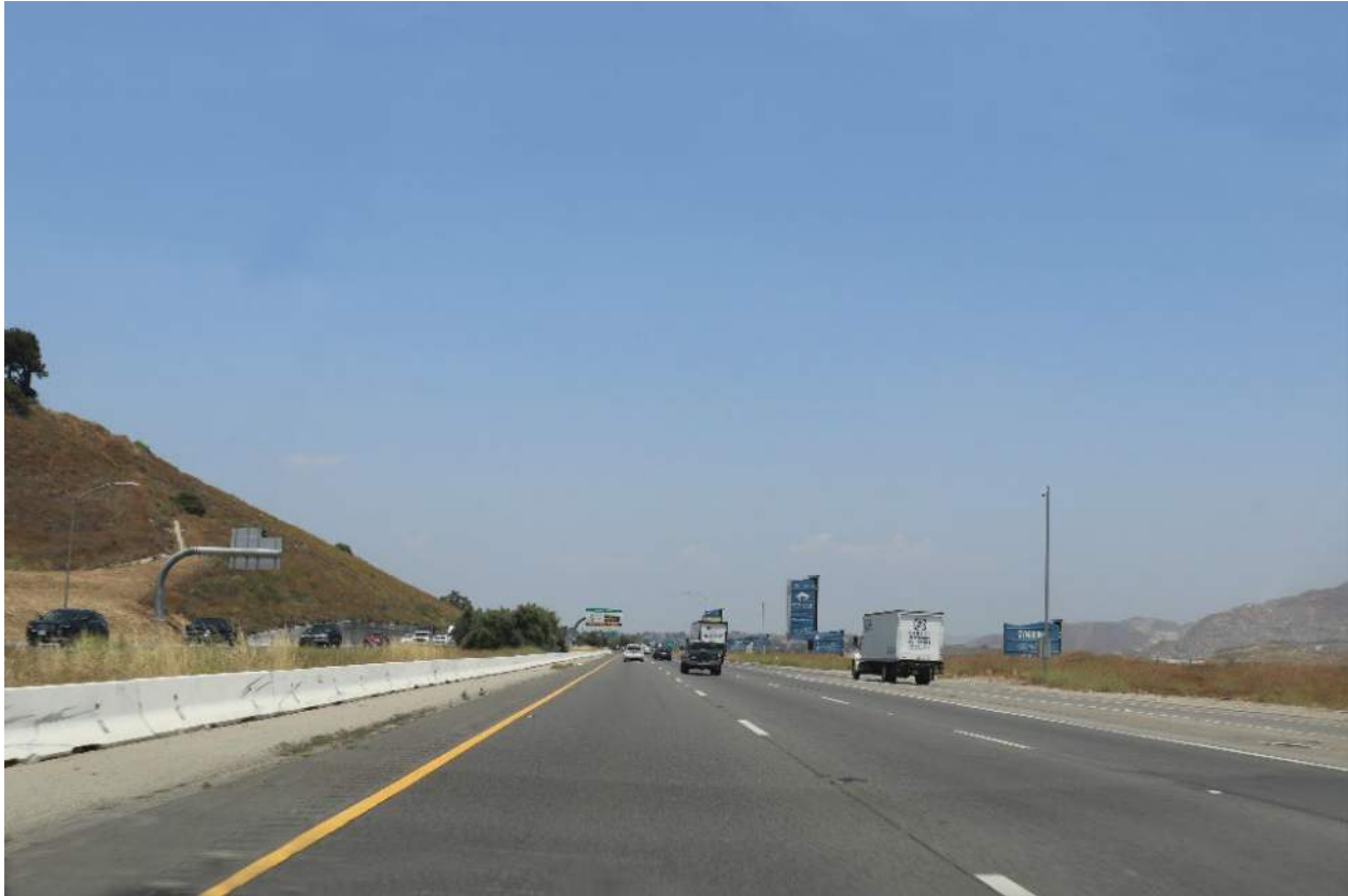
Figure 19. KV-5 Existing Condition
