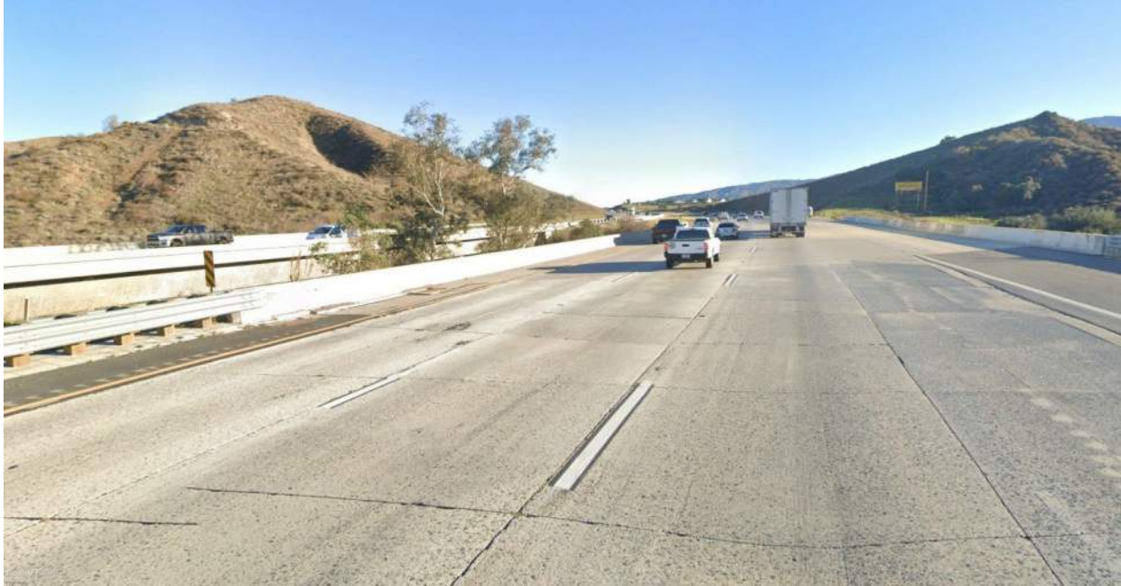
Figure 15a. KV-3a Existing Condition
