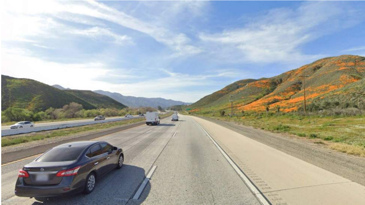
Figure 13. KV-2 Existing Condition
