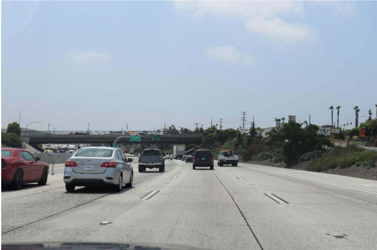
Figure 23. KV-7 Existing Condition
