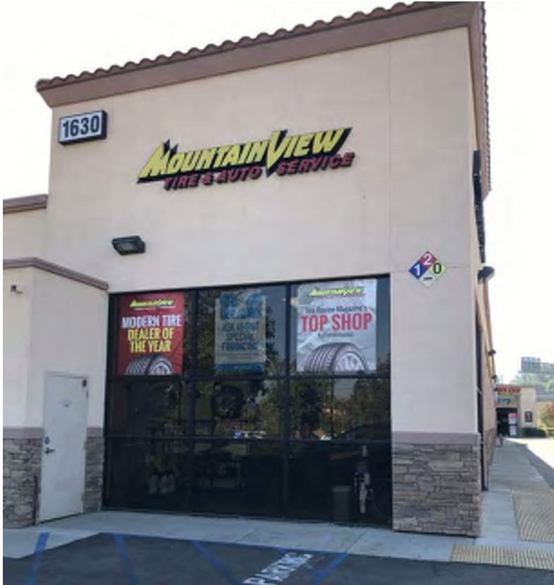
Site 102 – Mountain View Tire & Services Inc. (1630 E. Ontario Avenue, Corona, California). Photo facing south.
