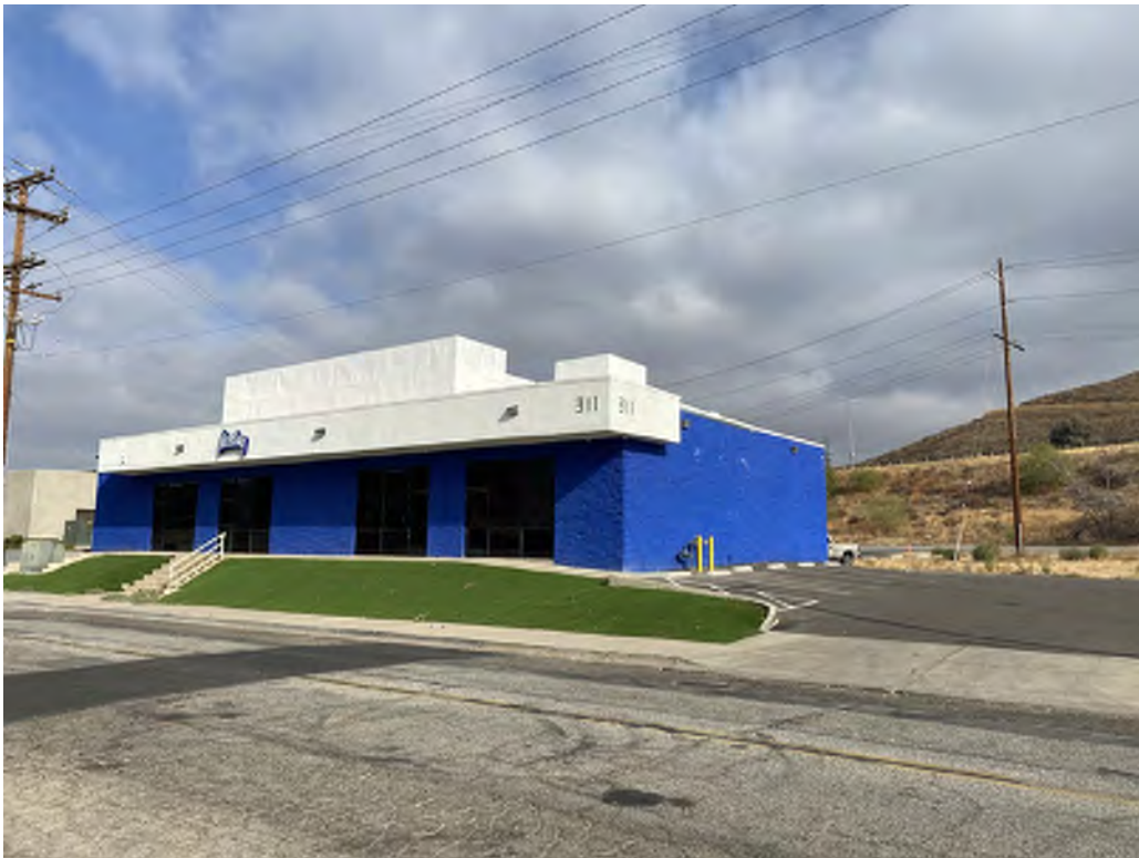
Site 9 – Abel's Auto Repair LLC (now Mr. Nice Guy) (311 W. Minthorn Street, Lake Elsinore, California). Photo facing northwest.
