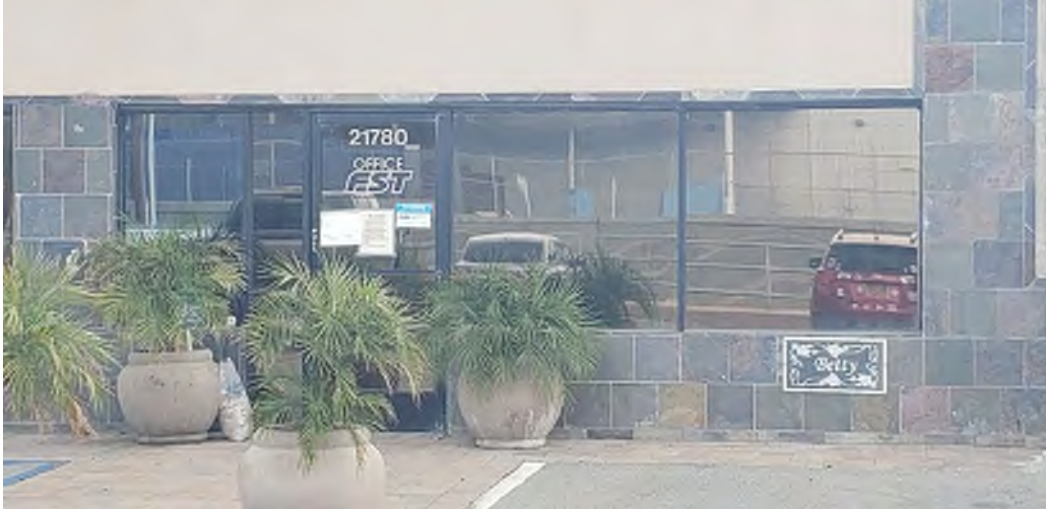
Site 72 – FST Sand & Gravel Inc. (21780 Temescal Canyon Road, Corona, California). Photo facing east.
