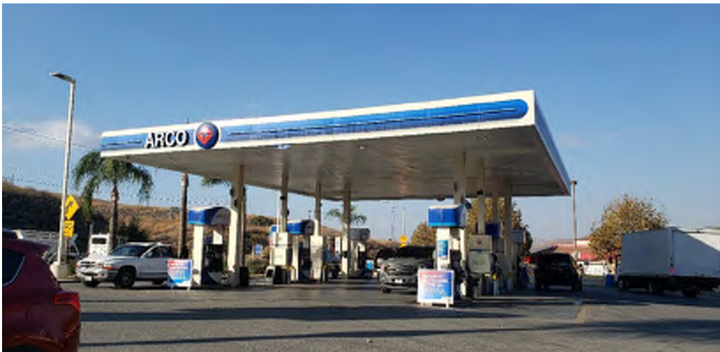
Site 54 – ARCO AM/PM Mini Mart (23760 Temescal Canyon Road, Corona, California). Photo facing northwest.
