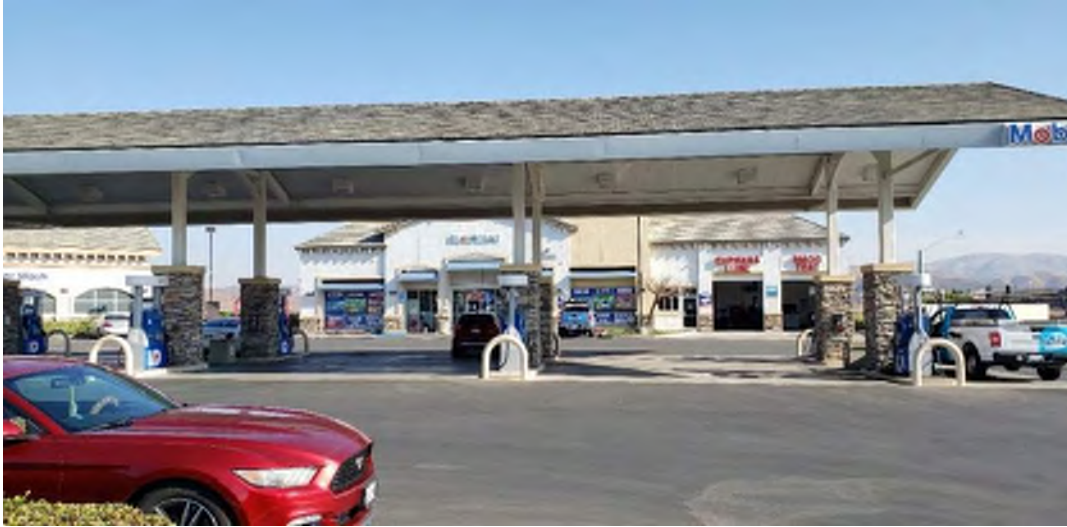
Site 81 – Eagle Glen Mobil LLC (2261 Eagle Glen Parkway, Corona, California). Photo facing east.
