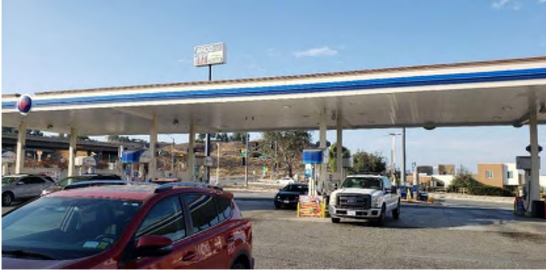
Site 74 – Dos Lagos ARCO (8765 Dos Lagos Dr, Corona, California). Photo facing northwest.
