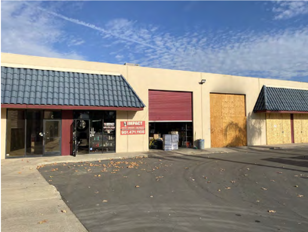
Site 14 – HI Tech Mechanical Services (now commercial business complex) (18650 Collier Avenue, Lake Elsinore, California). Photo facing northeast.
