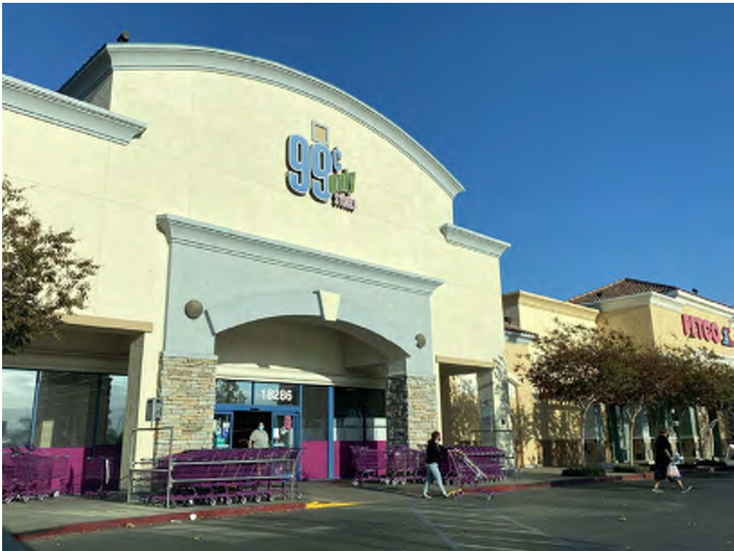
Site 23 – 99 Cents Only Store #234 (18286 Collier Avenue, Lake Elsinore, California). Photo facing northeast.
