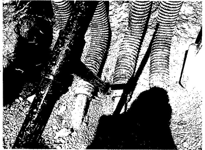
Existing manifold vent riser soil sampled due to vent lines being relocated.
