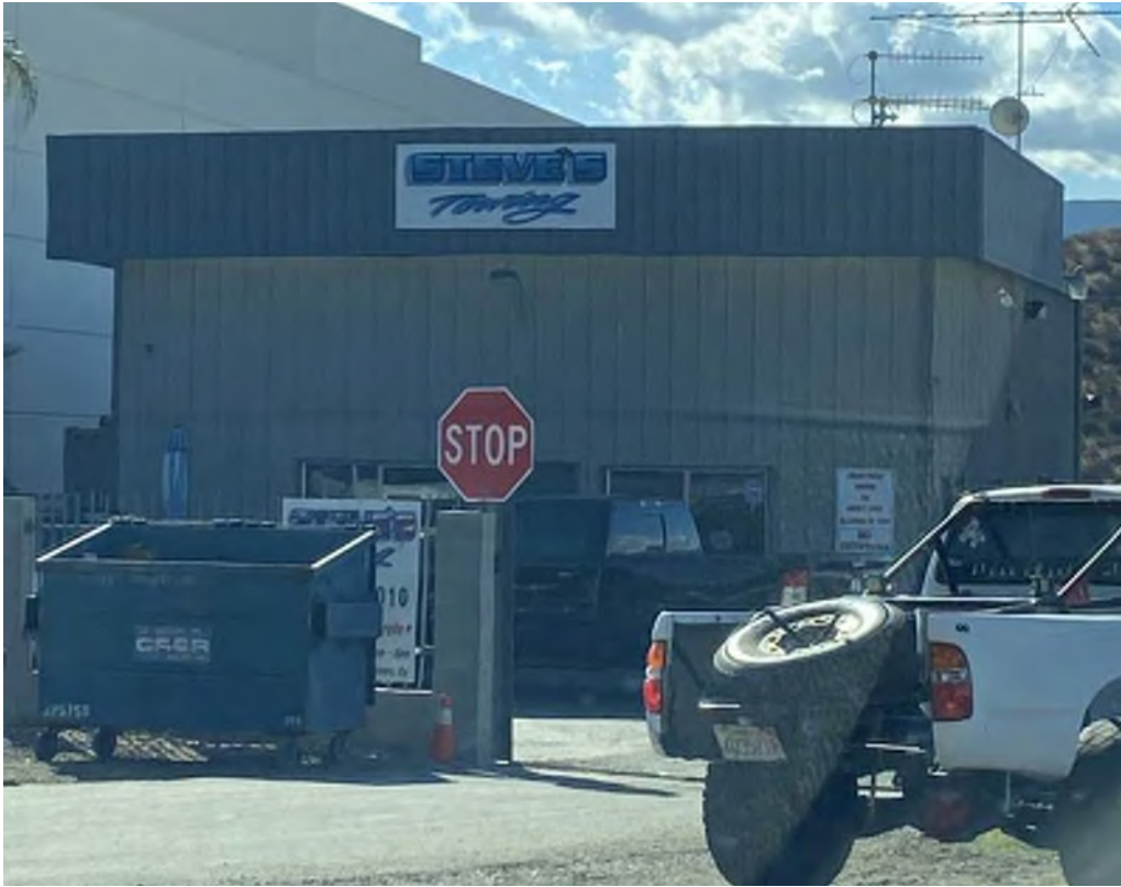
Site 10 – Laidlaw Transit (now Steve’s Towing) (609 Minthorn Street, Lake Elsinore, California). Photo facing southwest.
