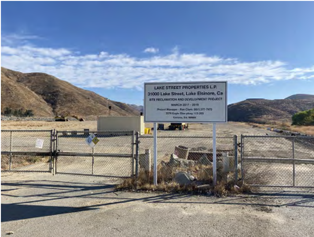
Site 35 – WYROC Lake Street Quarry (now vacant and for sale/lease property) (31000 Lake Street, Lake Elsinore, California). Photo facing east.
