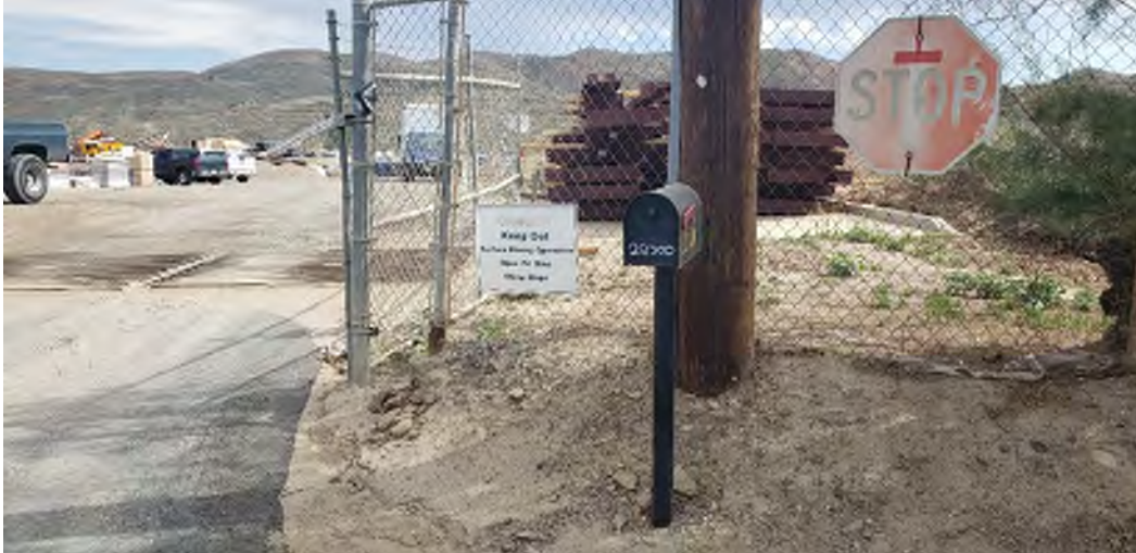
Site 68 – Standard Ready Mix Concrete (now Materials Specialties Corporation and Gail Materials) (22300 Temescal Canyon Road, Corona, California). Photo facing northeast.
