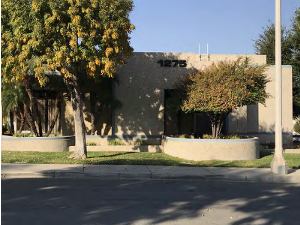
Site 112 – Advanced Fuel Filtration Systems (now South Coast Industrial Door) (1275 Graphite Drive, Corona, California). Photo facing north.
