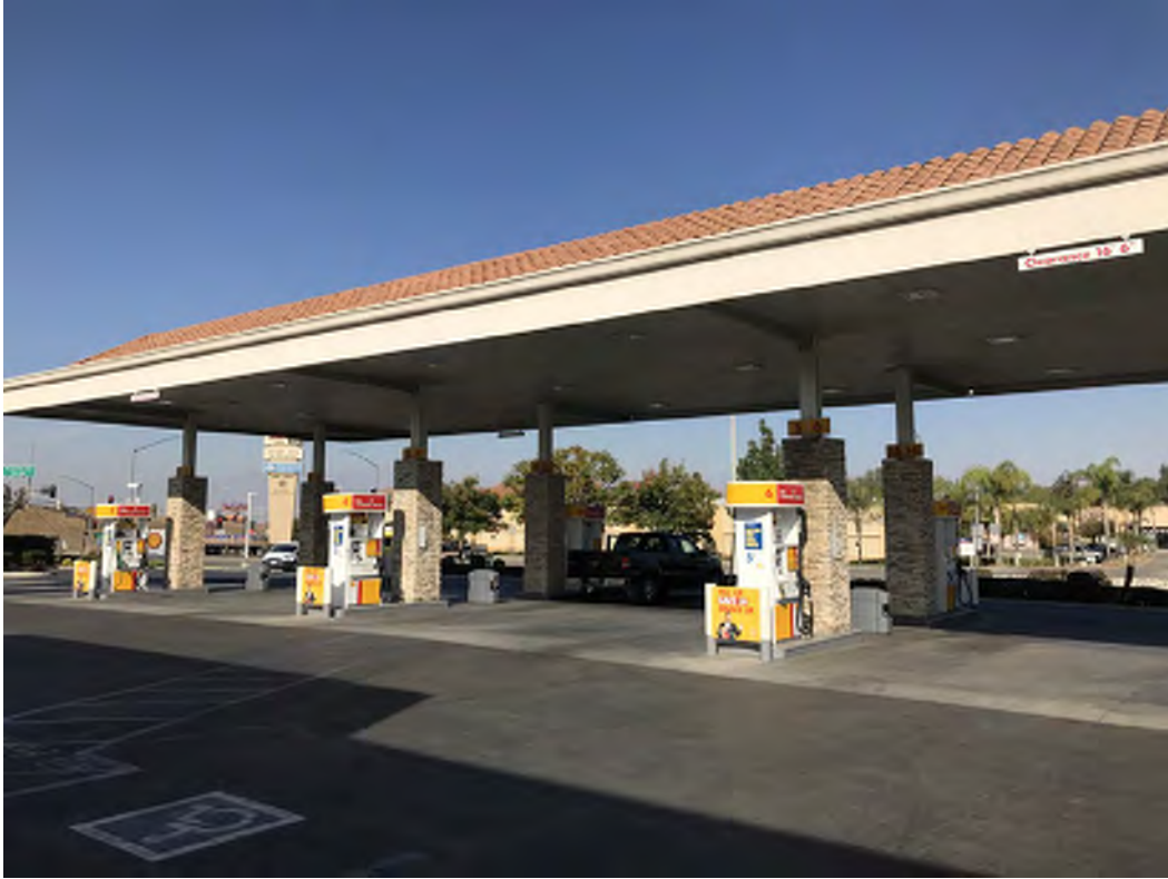
Site 104 – Corona Oil Co. Inc. / Shell (1550 E. Ontario Avenue, Corona, California). Photo facing north.
