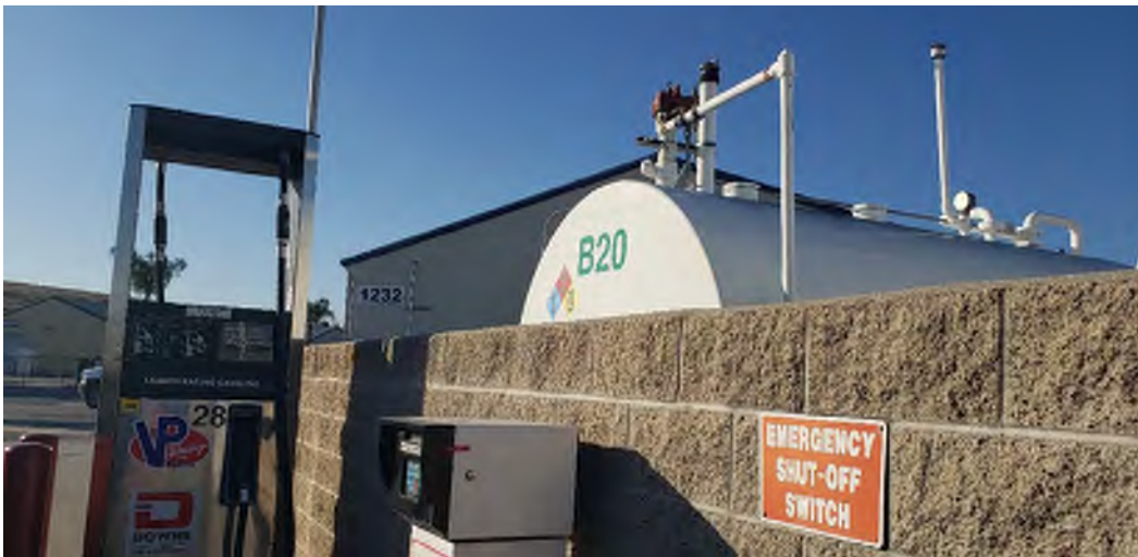
Site 123 – Downs Energy (1232 Magnolia Avenue, Corona, California). Photo facing south.
