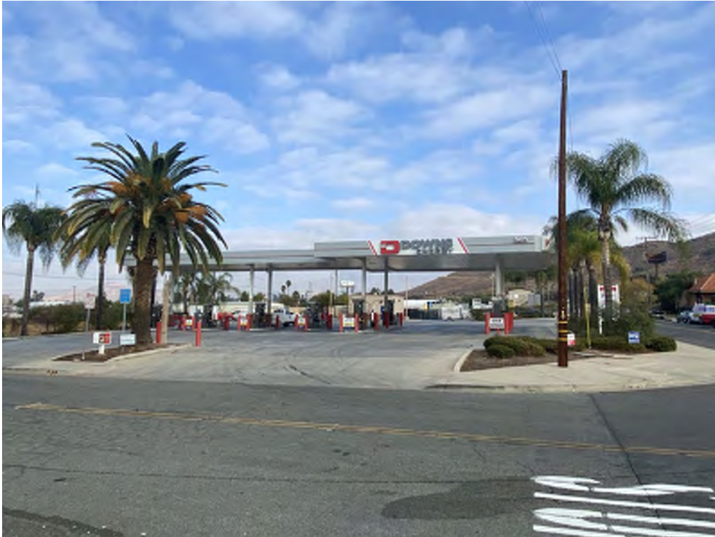
Site 5 – Big Al Oil Company (now Downs Energy) (501 Spring Street, Lake Elsinore, California). Photo facing north.
