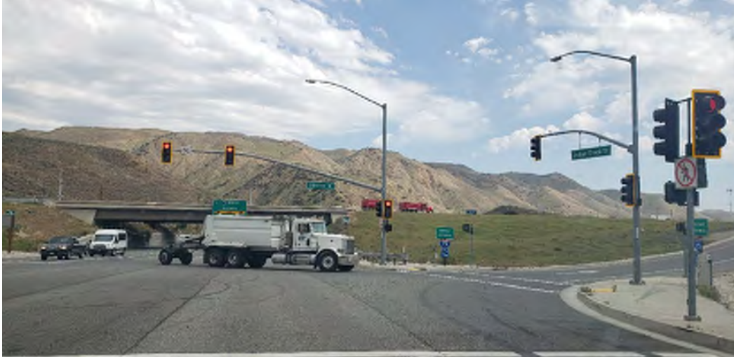
Site 49 – Indian Truck Trail I 15 Interchange (Temescal Canyon to Campbell Ranch Road, Lake Elsinore, California). Photo facing northeast.
