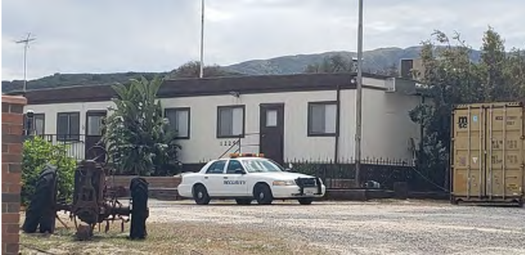
Site 45 – Hot Line Construction Inc. (12250 Temescal Canyon Road, Corona, California). Photo facing southeast.
