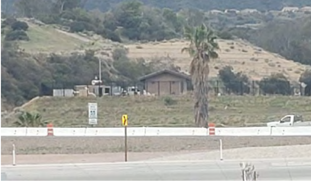
Site 77 – Arantine Hills Lift Station (2590 Bedford Canyon Road, Corona, California). Photo facing southwest.
