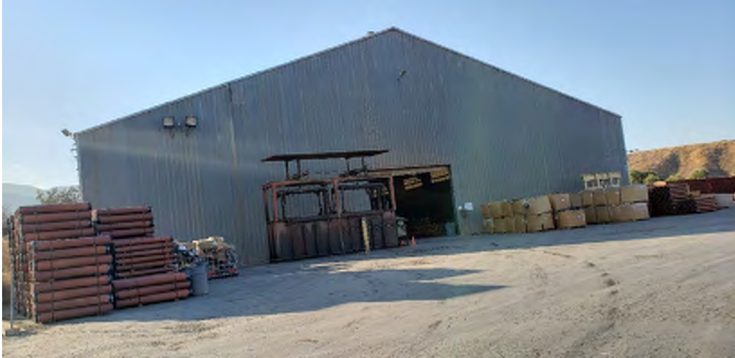
Site 53 – Mission Clay Products (23835 Temescal Canyon Road, Corona, California). Photo facing northwest.
