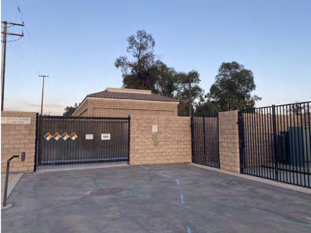
Site 16 – EVMWD-Rosetta I Pump Station (751 3rd Street, Lake Elsinore, California). Photo facing northeast.
