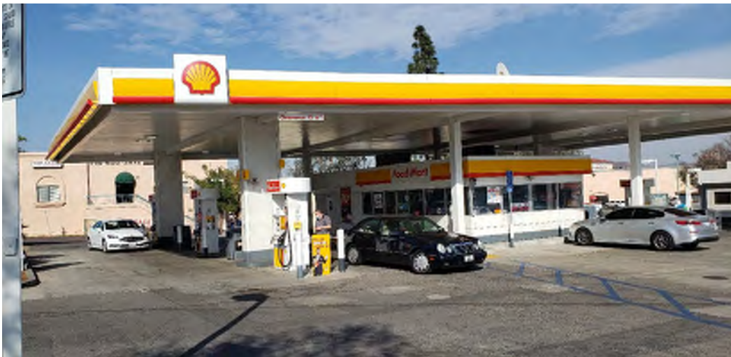
Site 121 – Shell Magnolia Corona (1205 Magnolia Avenue, Corona, California). Photo facing north.
