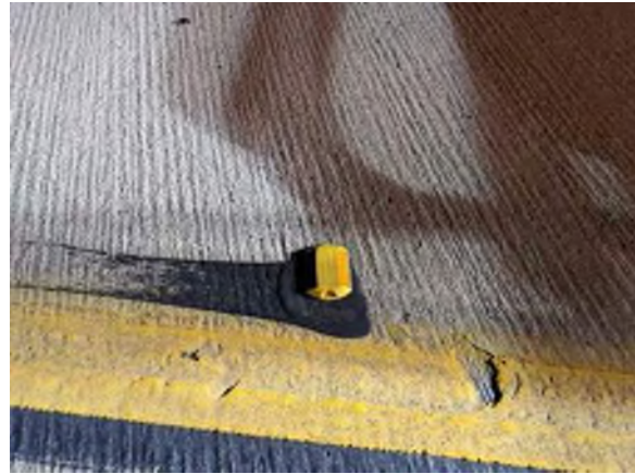
View of Yellow Lane Surface Paint on 56- 0677R – Northbound Indian Wash, Inside Rail
