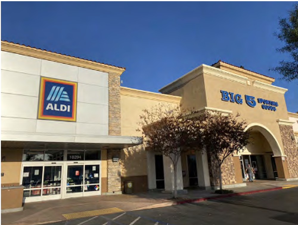
Site 21 – ALDI Inc. DBA ALDI #78 (18294 Collier Avenue, Lake Elsinore, California). Photo facing northeast.
