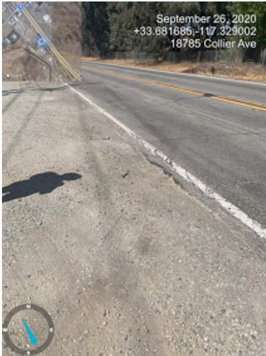
Photo 13: Feature 6008. Photo taken looking northwest.
