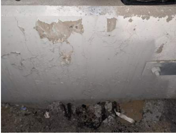
View of Light Gray Paint on 56-0680R – Northbound Temescal Wash, Inside Rail
