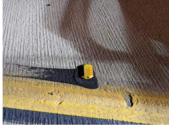
View of Yellow Lane Surface Paint on 56- 0677R – Northbound Indian Wash, Inside Rail
