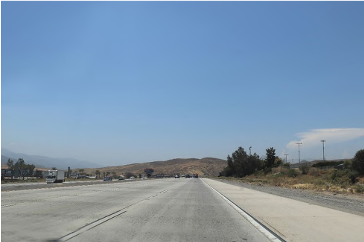
Figure 2.2.9-2. KV-1 Existing Condition
