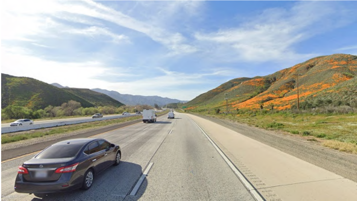
Figure 2.2.9-4. KV-2 Existing Condition
