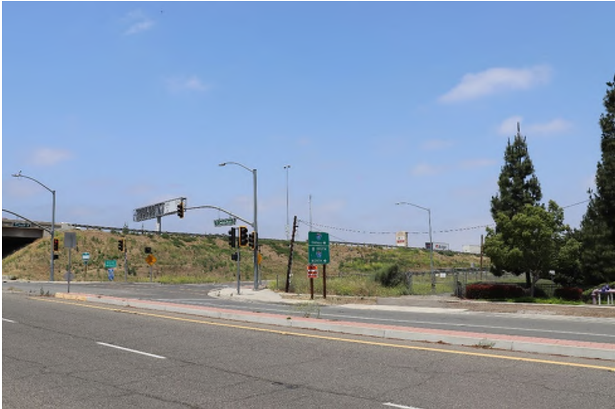
Figure 2.2.9-14. KV-6 Existing Condition
