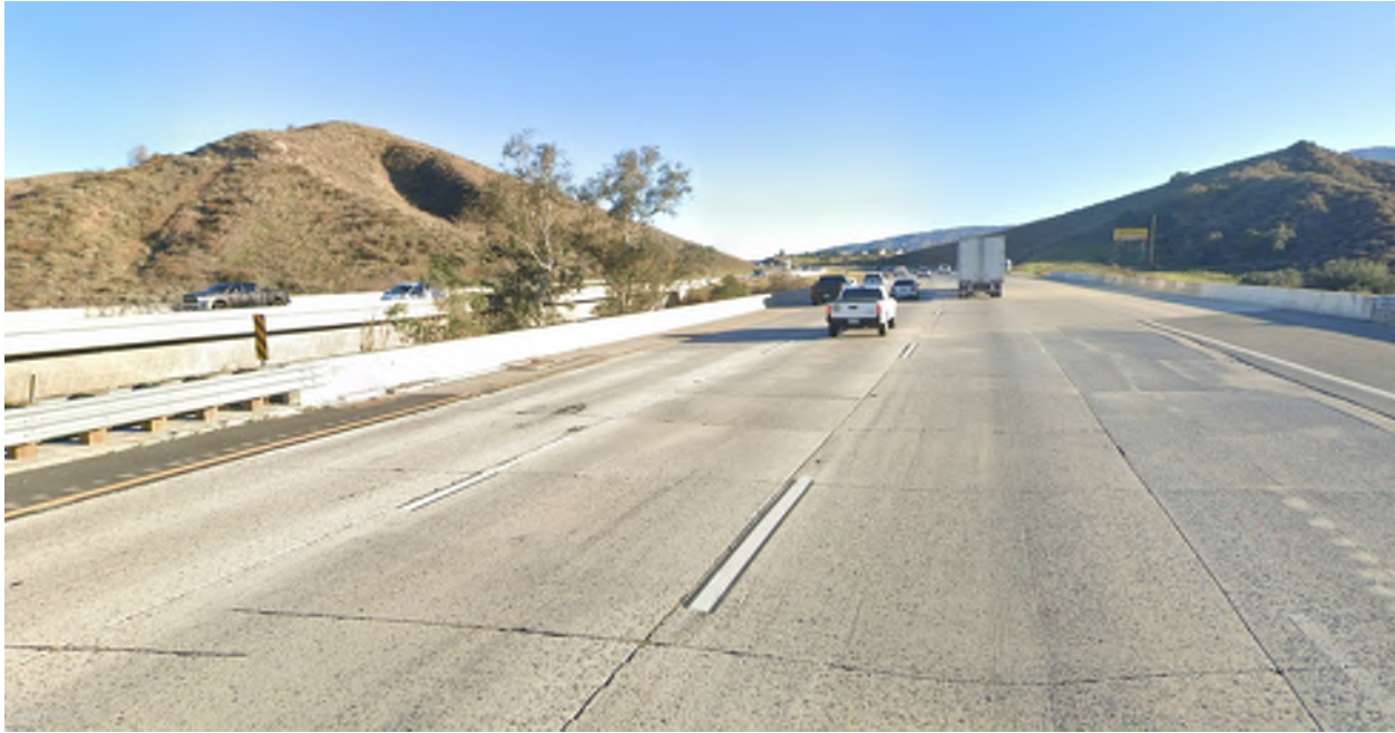
Figure 2.2.9-6. KV-3a Existing Condition
