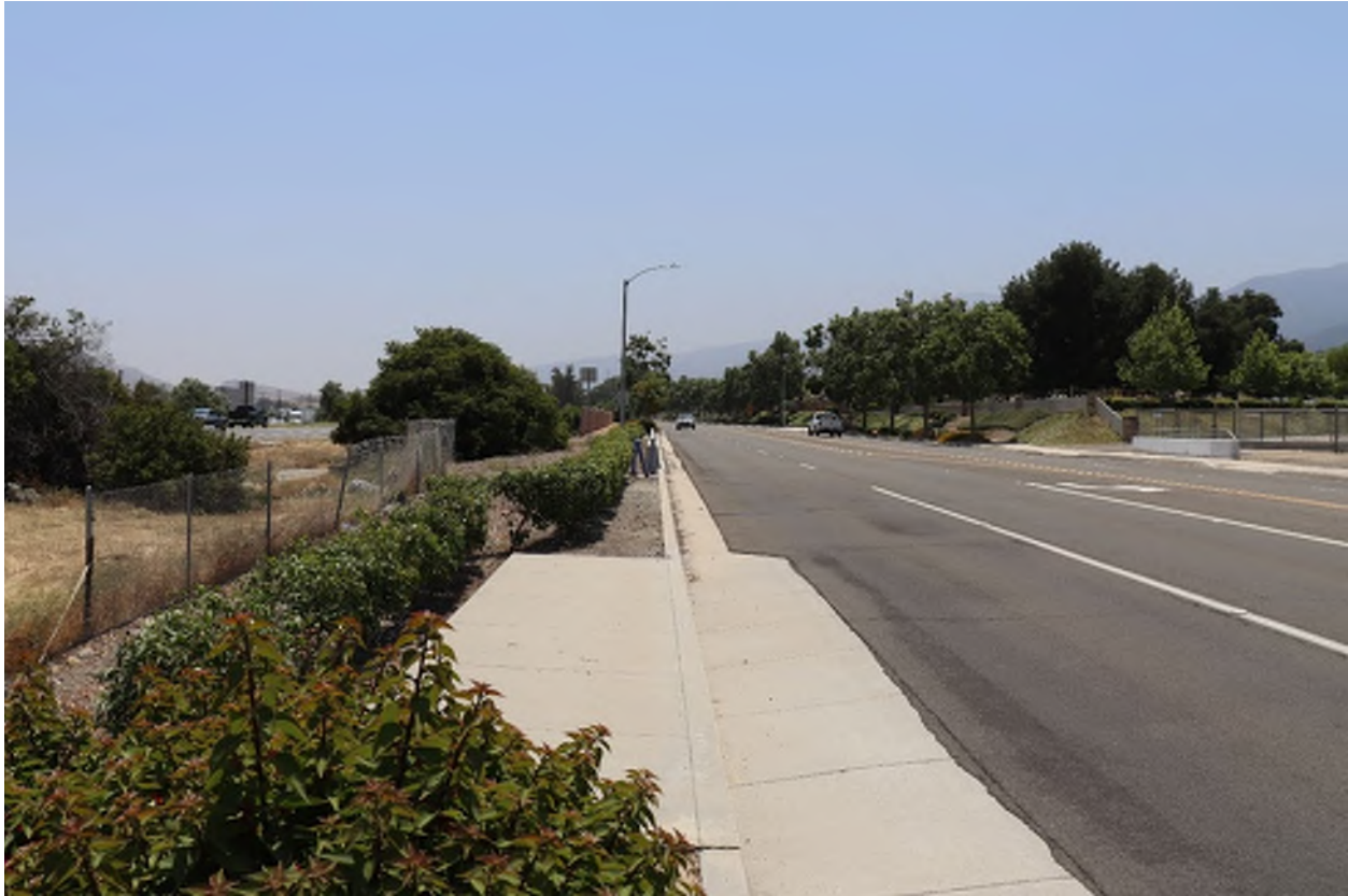
Figure 2.2.9-10. KV-4 Existing Condition
