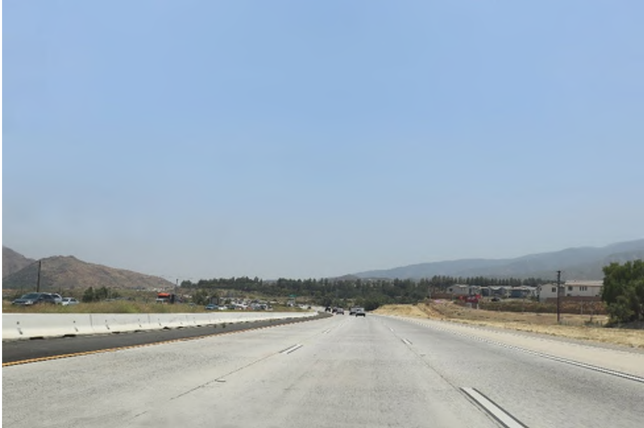
Figure 2.2.9-8. KV-3b Existing Condition
