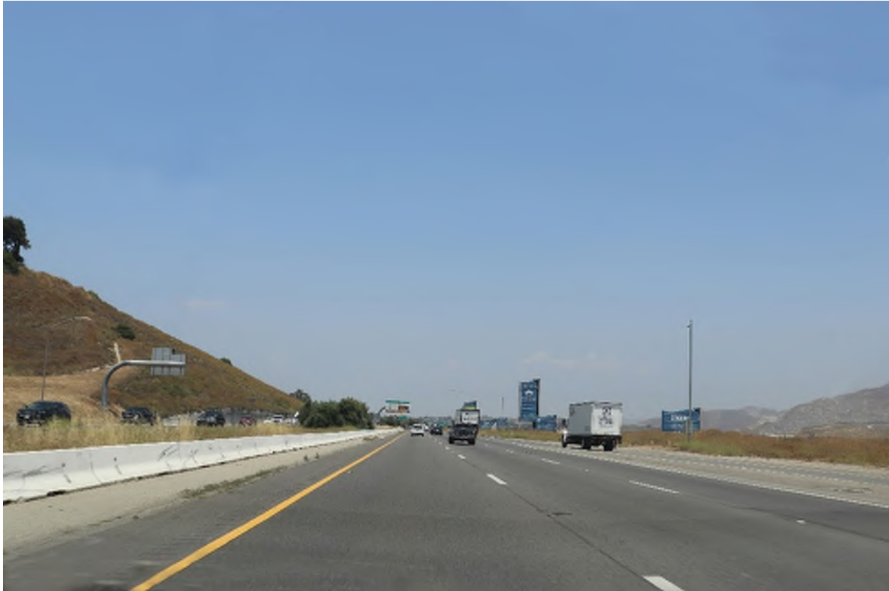
Figure 2.2.9-12. KV-5 Existing Condition
