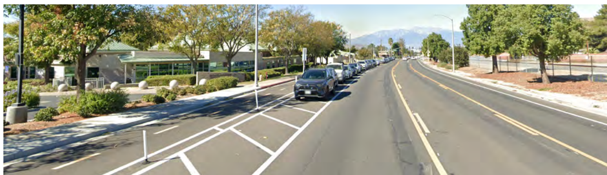
PROTECTED BIKE LANES (WATKINS DRIVE) SOURCE: GOOGLE EARTH
