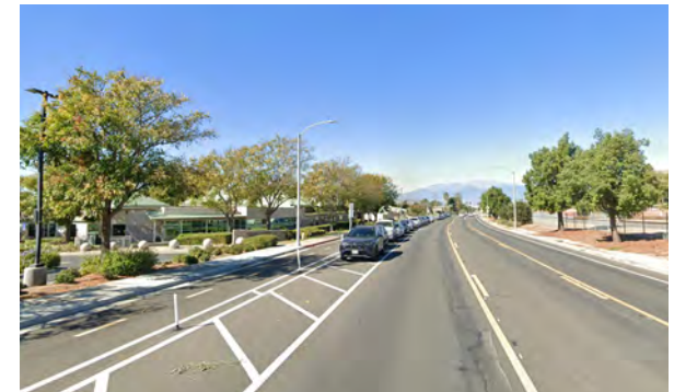
PROTECTED BIKE LANES (WATKINS DRIVE) SOURCE: GOOGLE EARTH
