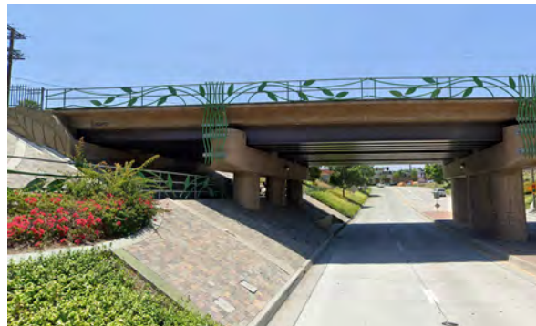
UNDERPASS IMPROVEMENTS SOURCE: GOOGLE EARTH
