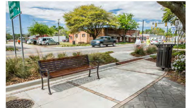
ROADWAY WITH PEDESTRIAN INFRASTRUCTURE
