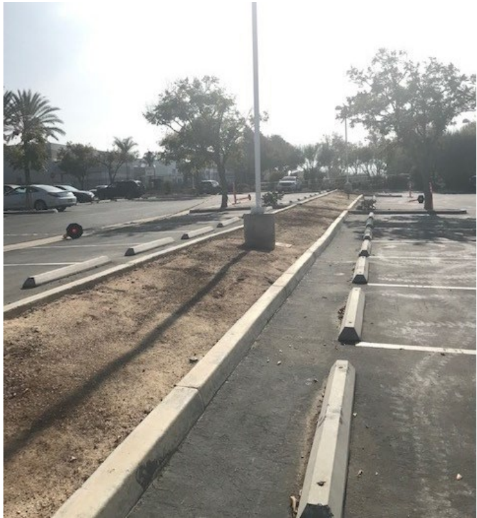
Corona - West Station - BEFORE
