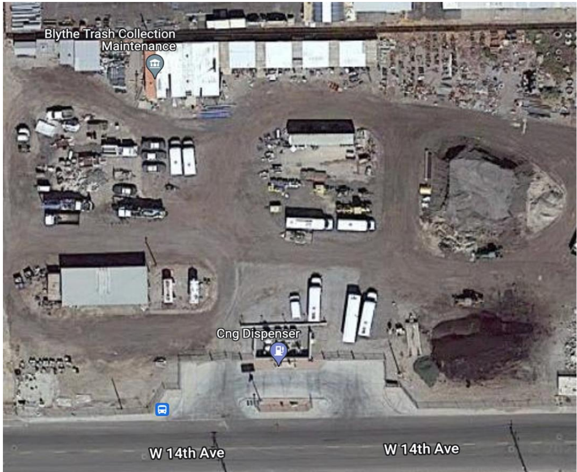
Figure 4 - Facilities Overview: CNG fueling Station
