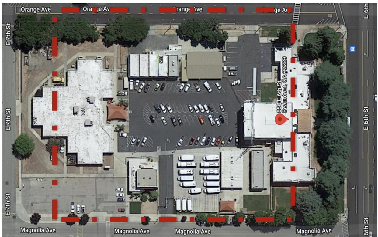
Figure 3 – Administrative Facility Overview
