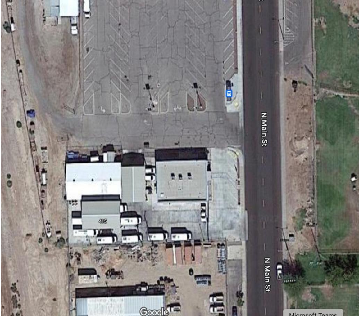
Figure 3 – Facilities Overview: Administrative and Maintenance
